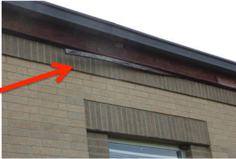
Photo 55 One piece of wood trim was loose...
