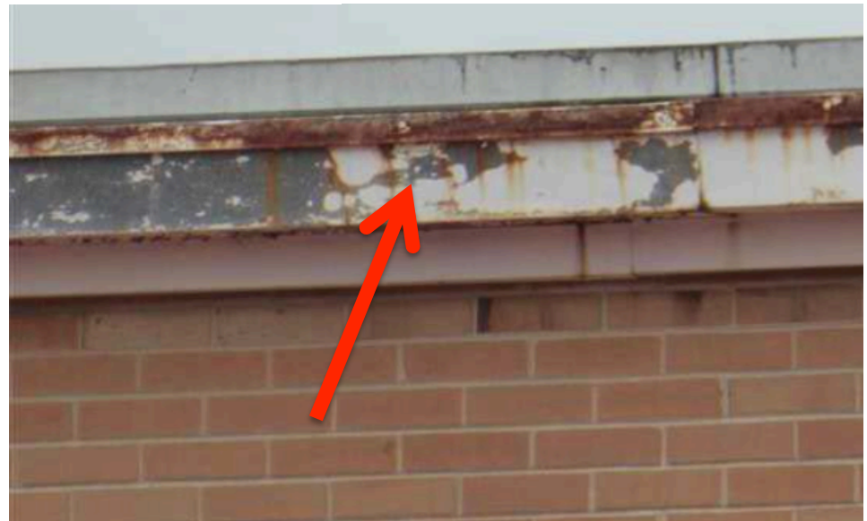
Photo 20 Peeling paint has left the metal exposed allowing it to corrode.
